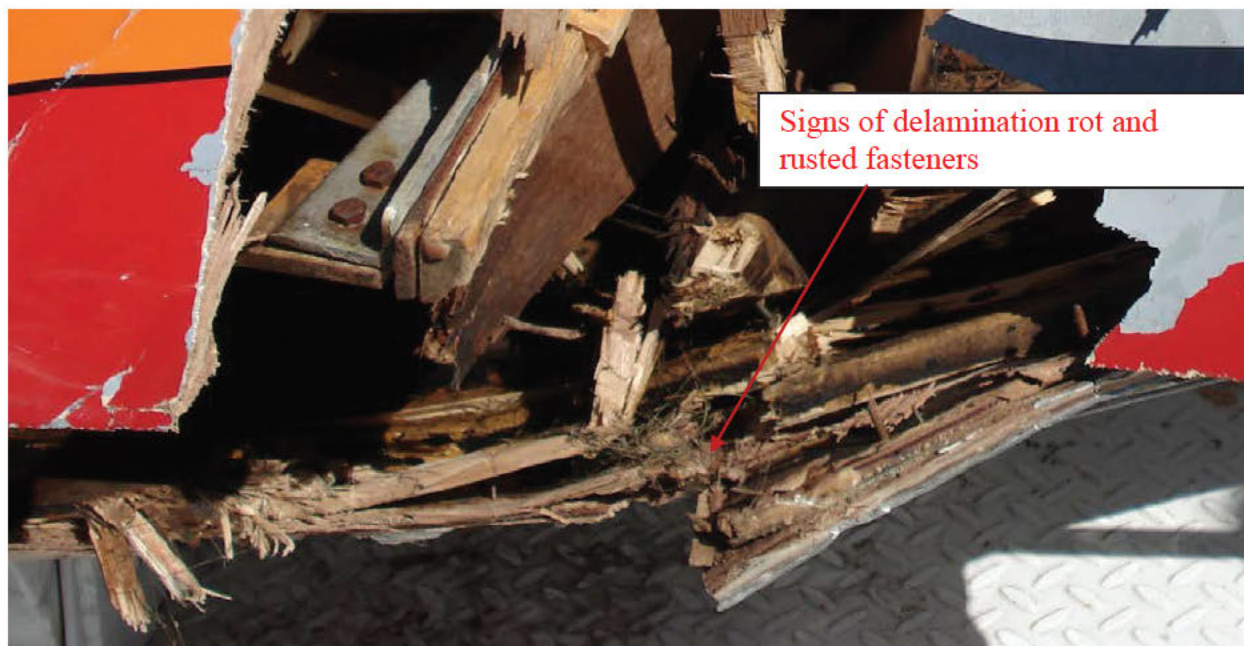
Figure 15 – Close up image of the damage to the GNH-12 indicated signs of delaminating, rot, and rusted fasteners
